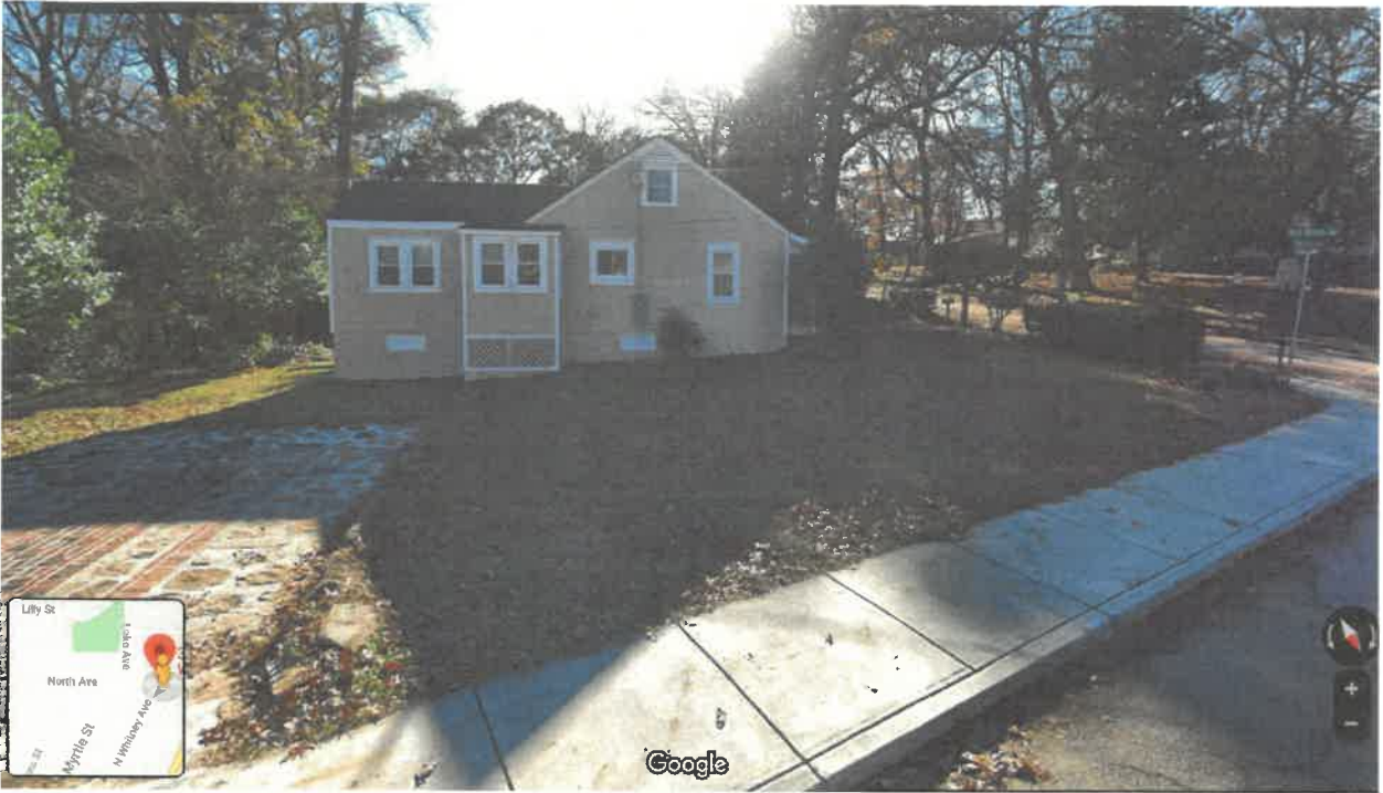
Left Side Elevation Prior to Addition
