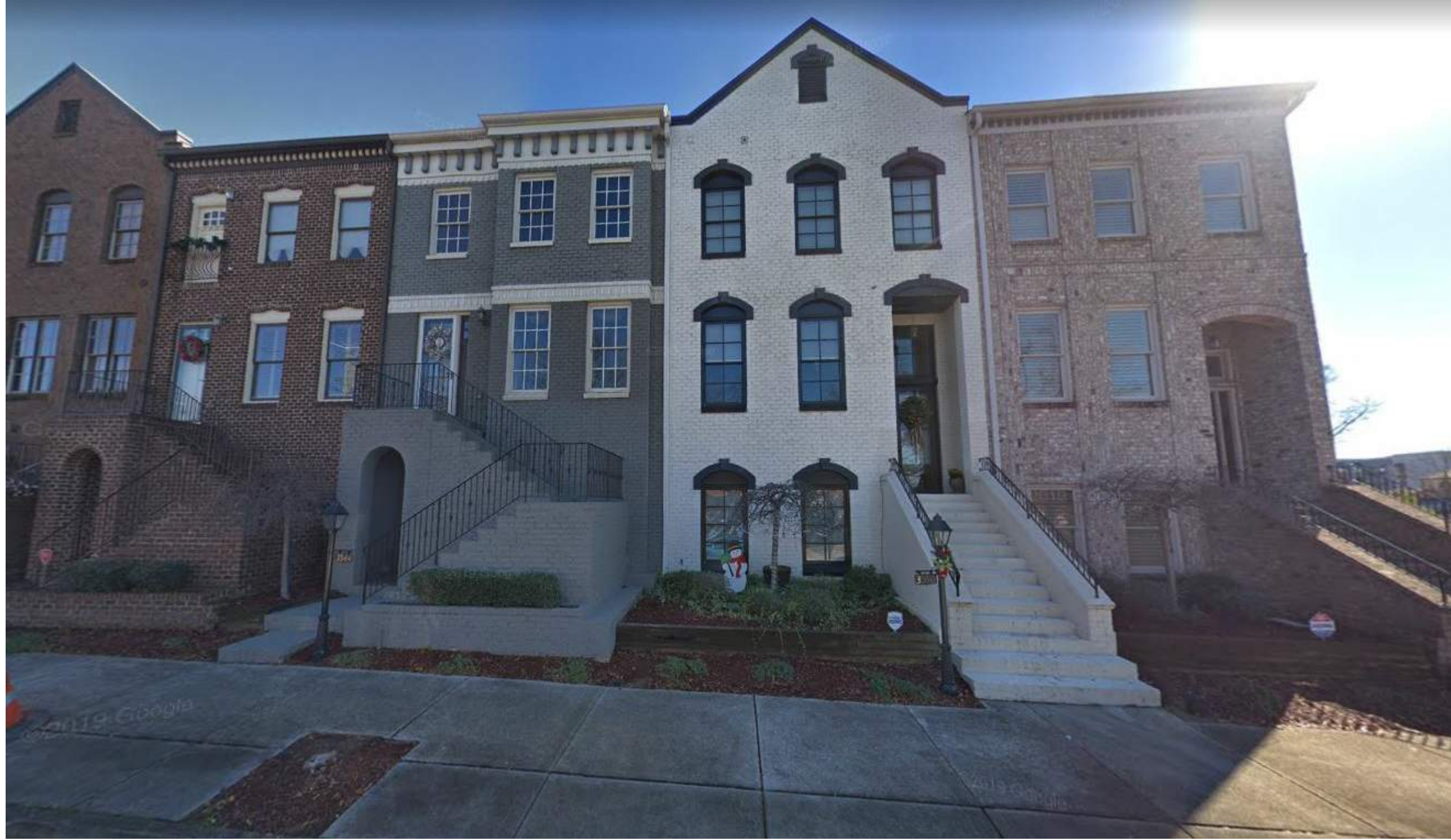
NEIGHBORING PROPERTY HAS LOWER SLOPE ROOFS THAT APPEAR FLAT FROM THE STREET
