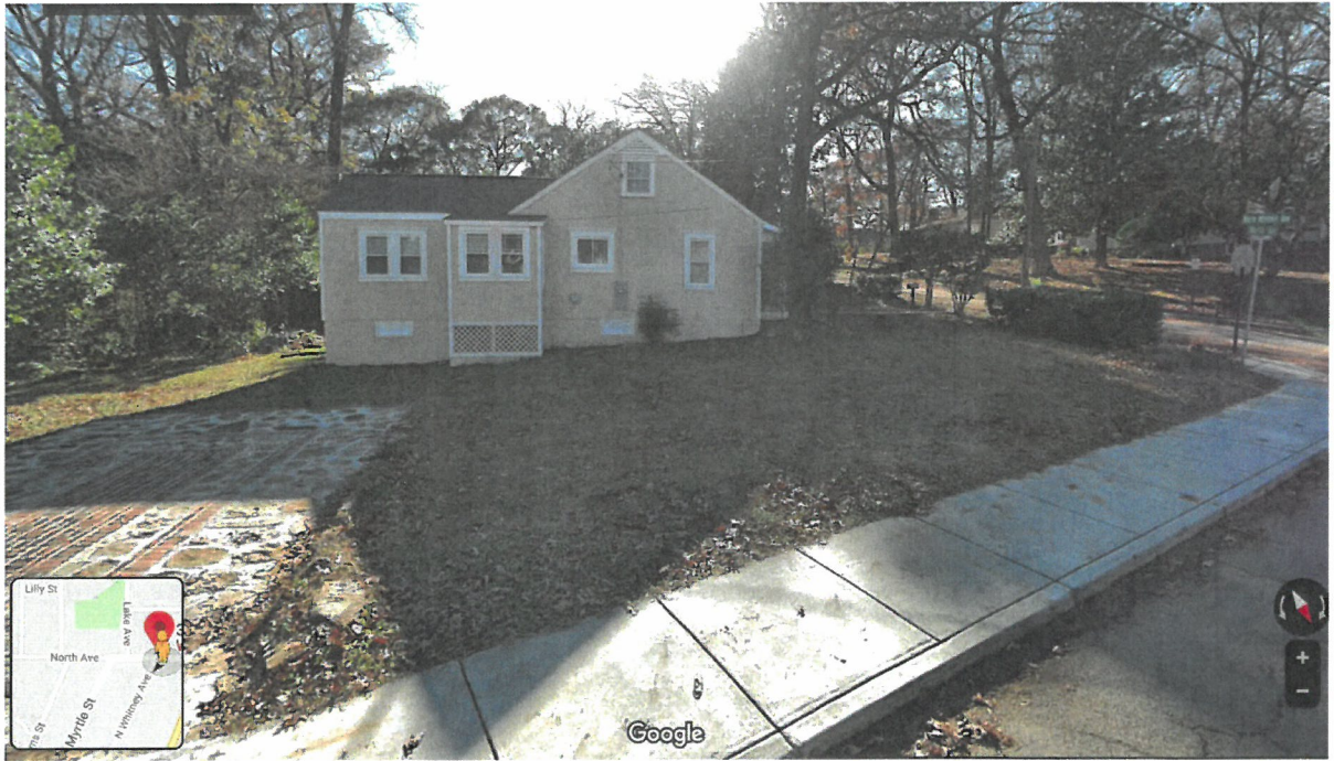
Left Side Elevation Prior to Addition
