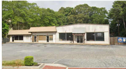
CURRENT BUILDING PHOTO
