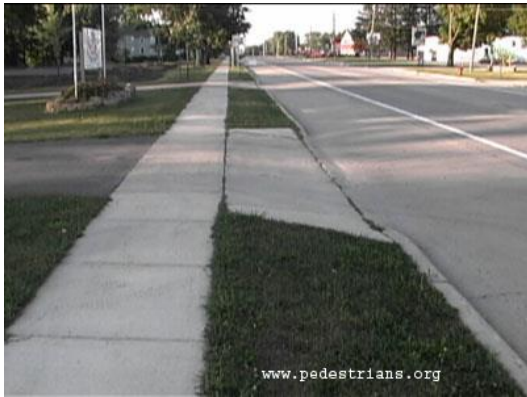
Figure 1 – Continuous sidewalk material
