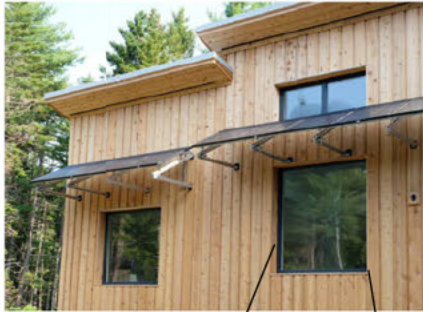
EXTERIOR CLADDING AND WINDOW TRIM CONCEPT IMAGE
