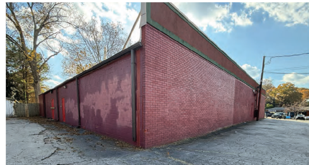
Back corner of building facing North Ave.
