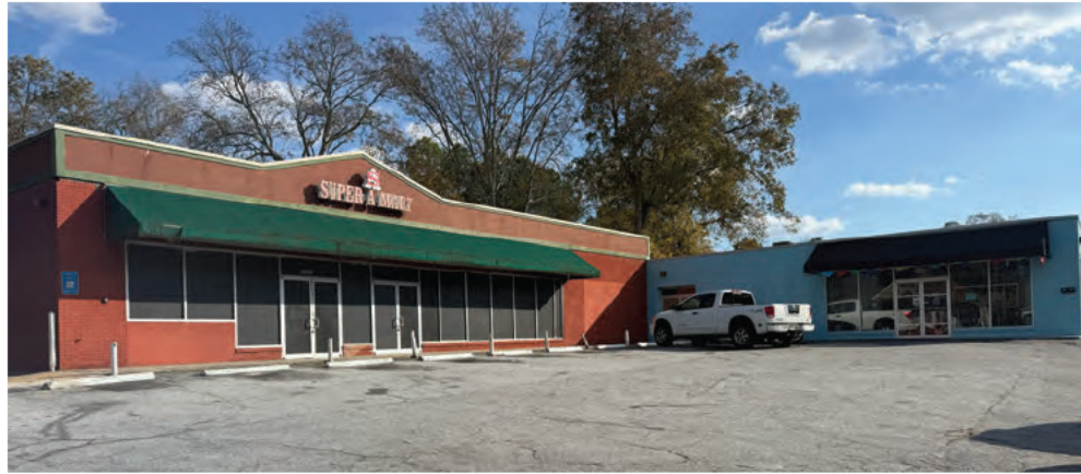
Front corner of building facing Dogwood / North Ave. intersection
