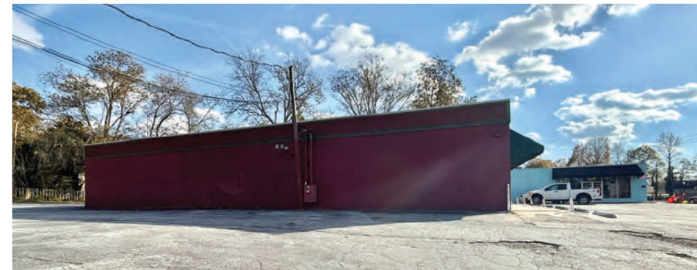
Side of building facing North Ave.
