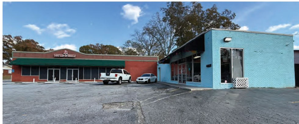
Front of building facing Dogwood Drive
