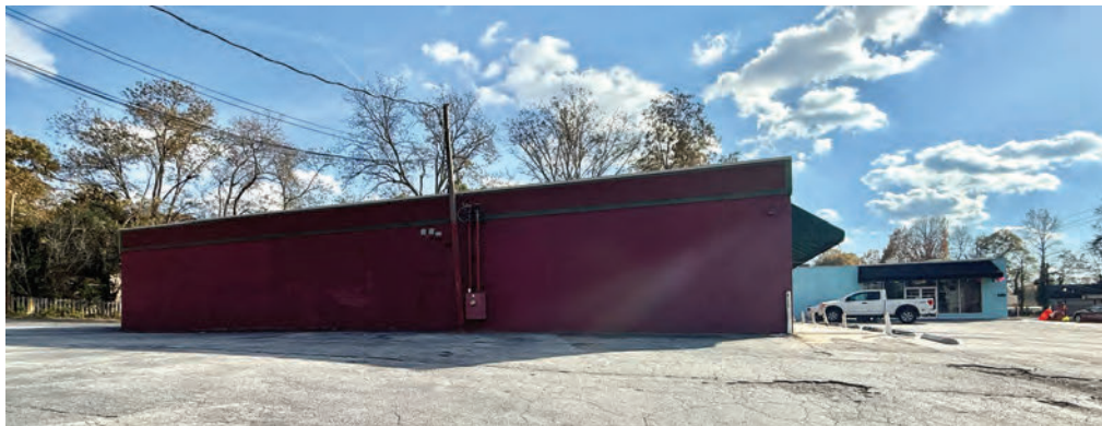
Side of building facing North Ave.
