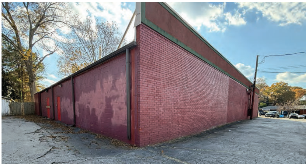
Back corner of building facing North Ave.
