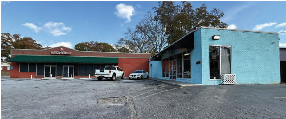
Front of building facing Dogwood Drive
