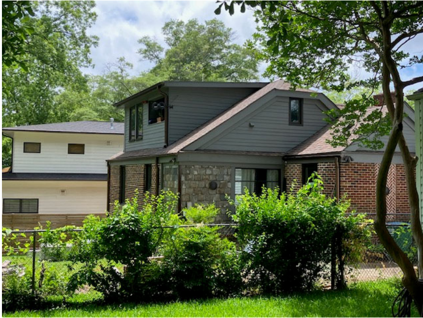
NORTH SIDE VIEW AND BACK VIEW
