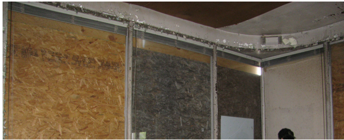
INTERIOR CURVED STOREFRONT CORNER
