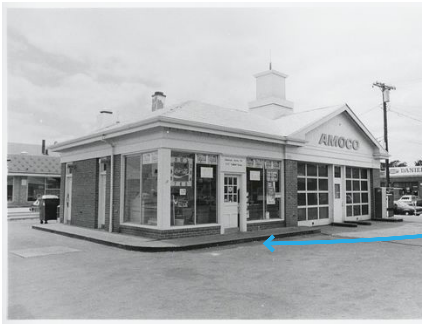
1970'S AMOCO GAS STATION RENOVATION
