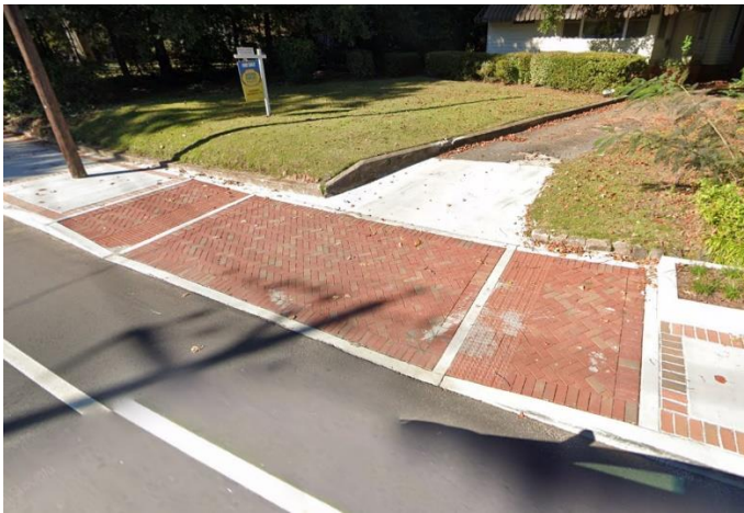
Figure 2 – Brick pavers across a driveway
