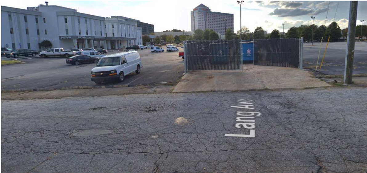
EXISTING TRASH ENCLOSURE (EAST STREET VIEW)
