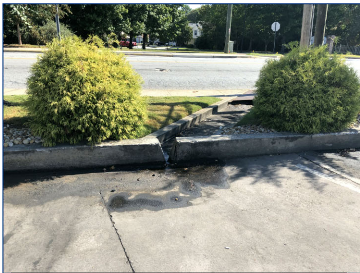
13 - Flume Near Refuse Enclosure
