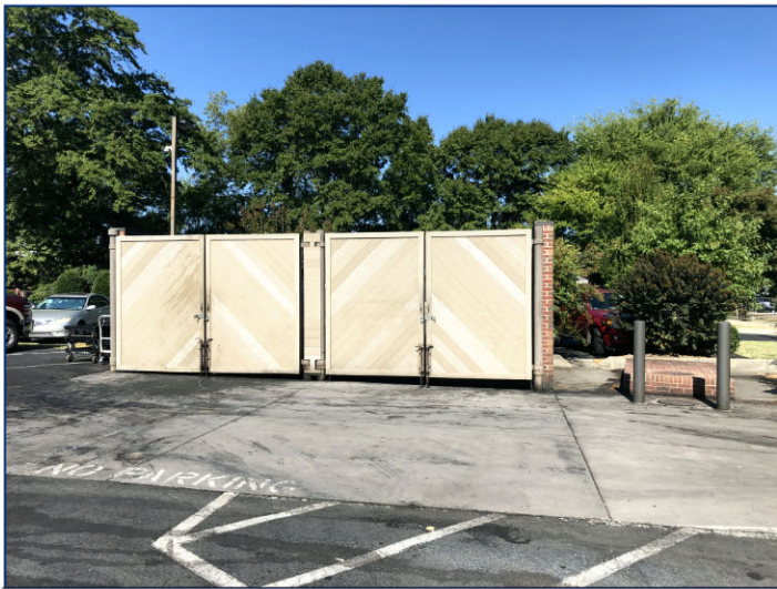
11 - Refuse Enclosure & Grease Trap
