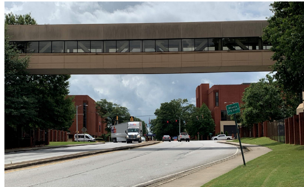
LOOKING SOUTH ALONG DELTA BOULEVARD TOWARDS NORTH OUTER LOOP ROAD.
