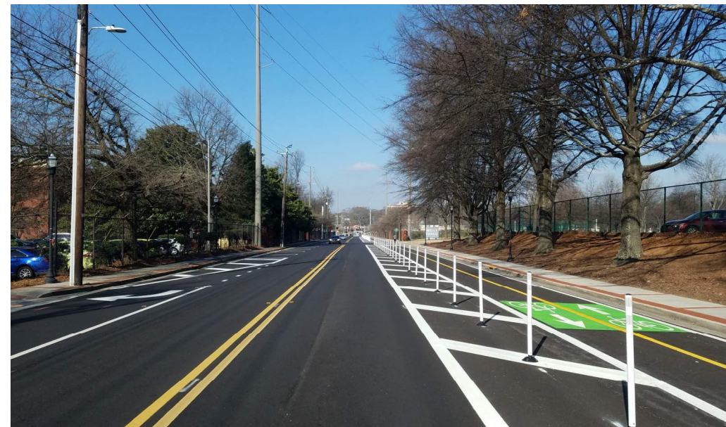
EXISTING CYCLE-TRACK LOOKING NORTH-WEST ALONG DOUG DAVIS DRIVE
