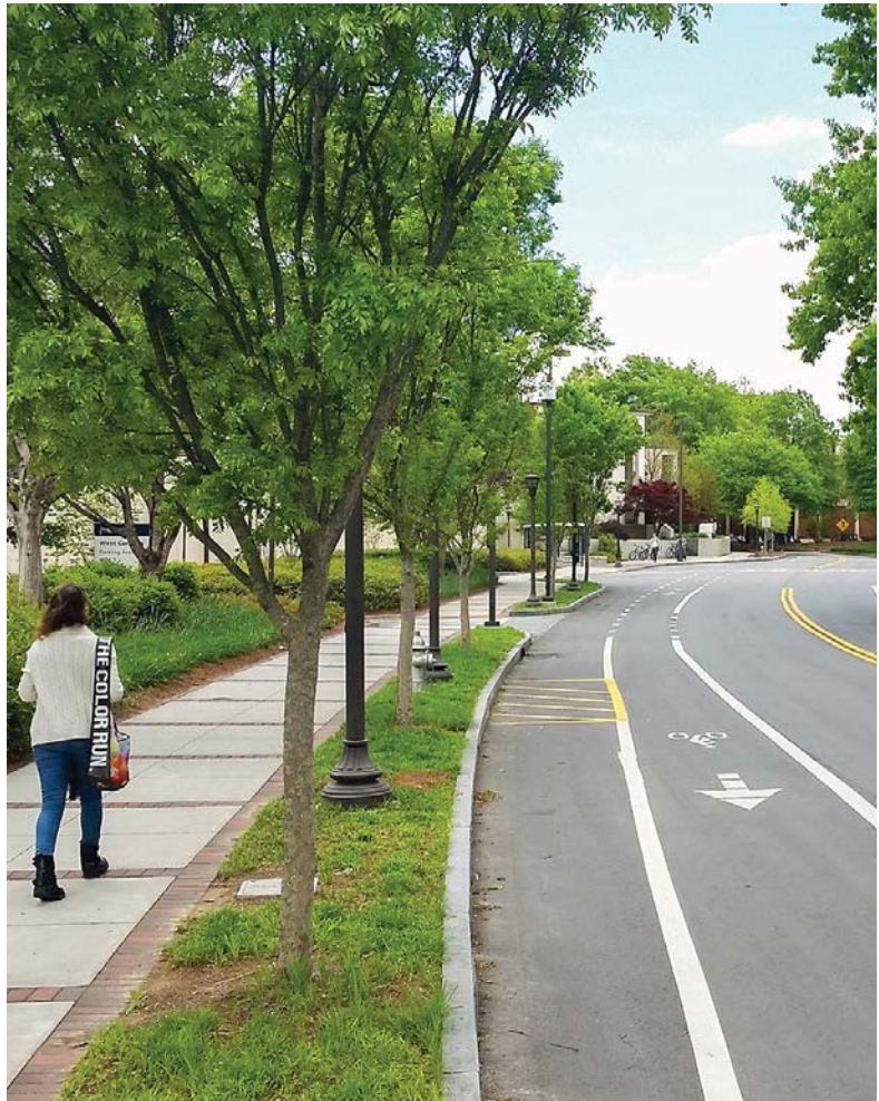
Example of a landscape strip that provides separation between a pedestrian path and vehicular traffic on Georgia Tech's campus.
