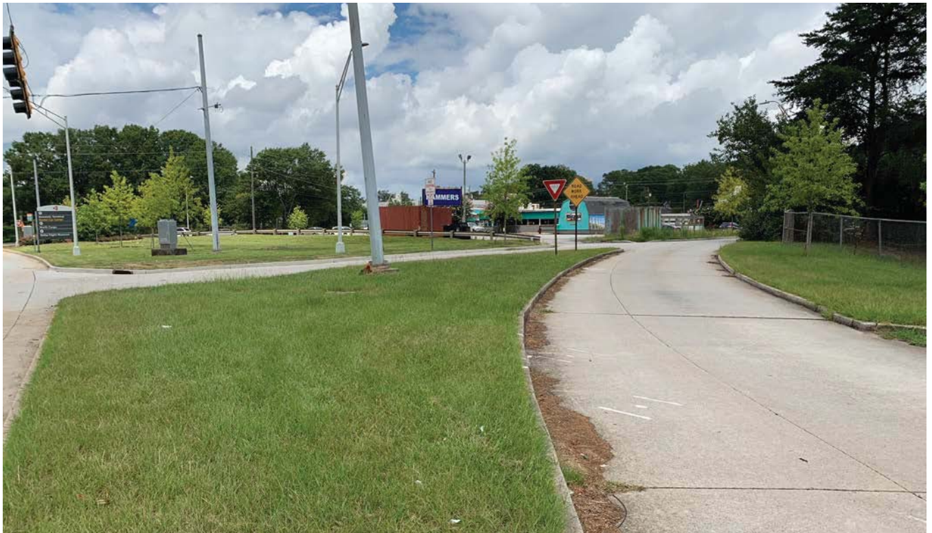
Existing conditions of the slip lane looking north to Oakridge Avenue.
