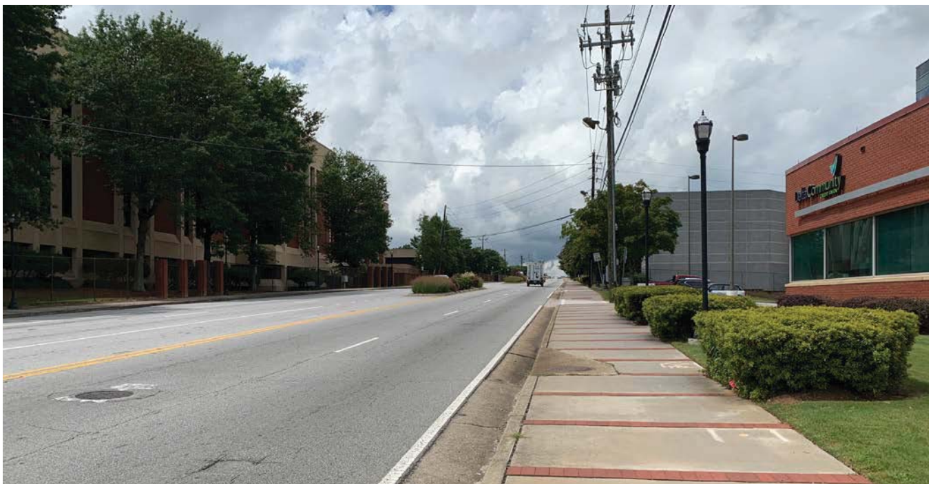
Existing conditions on Virginia Avenue looking west toward Delta Boulevard.
