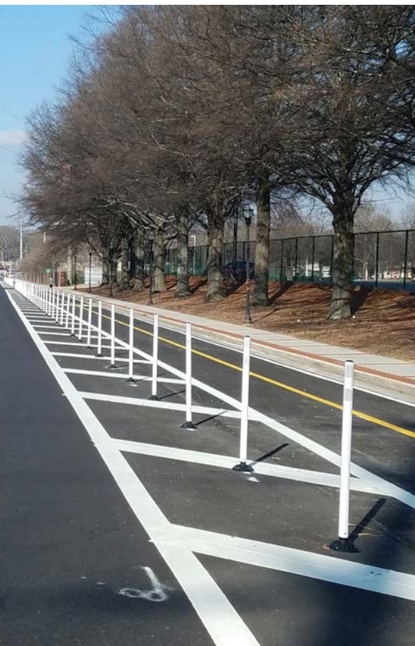
View of the cycle track along Doug Davis Drive. This is a potential connection opportunity for the model mile and would create a more expansive bike network within the study area.
