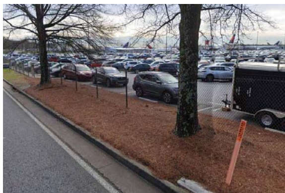
The fiber optic cable running through a portion of the study area, indicated by this marker adjacent to North Inner Loop Road, will need to be protected during construction of the model mile.
