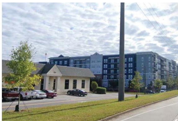
Existing transmission line power poles adjacent to Perry J Hudson Parkway are to be avoided if the model mile terminus extends further east past the site.
