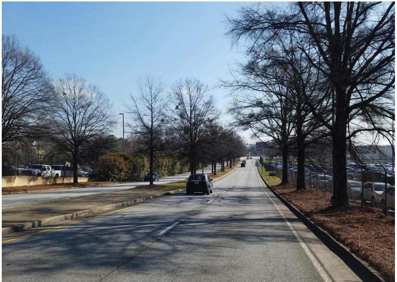
Existing conditions present on North Inner Loop Road (looking east) adjacent to an airport parking lot.
