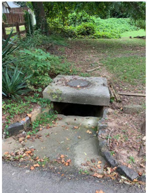
Existing Storm Catch Basin along Lake Avenue
