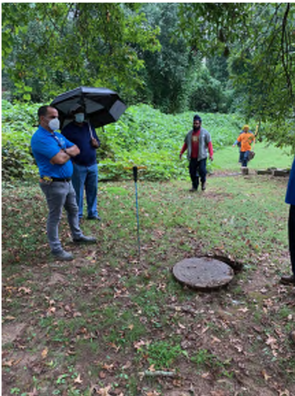
Existing Sewer Manhole Tie-In Location on Adjacent Property along Lake Avenue
