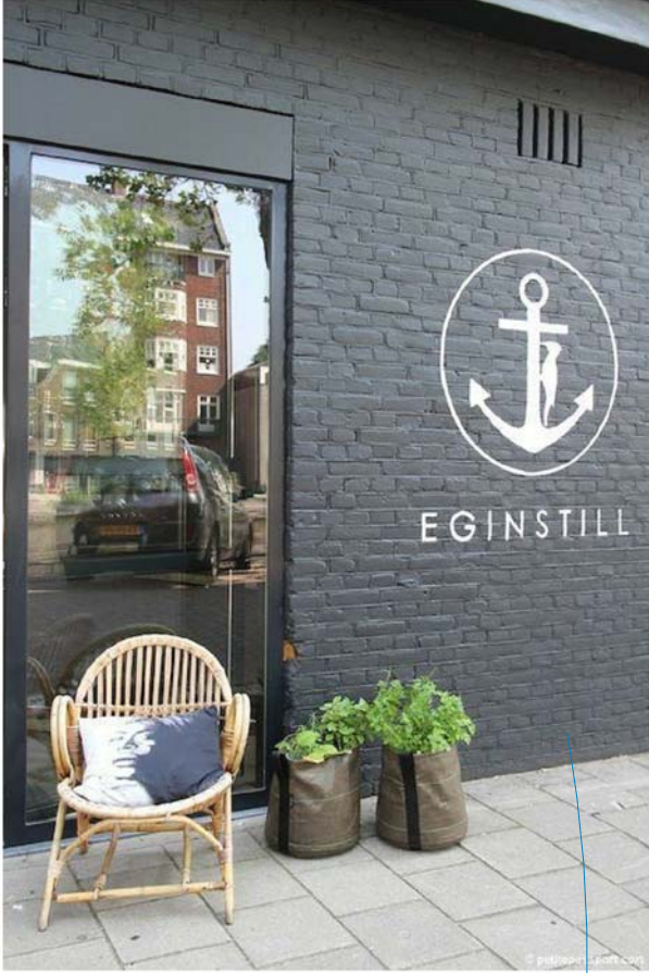
PAINTED BRICK FACADE
