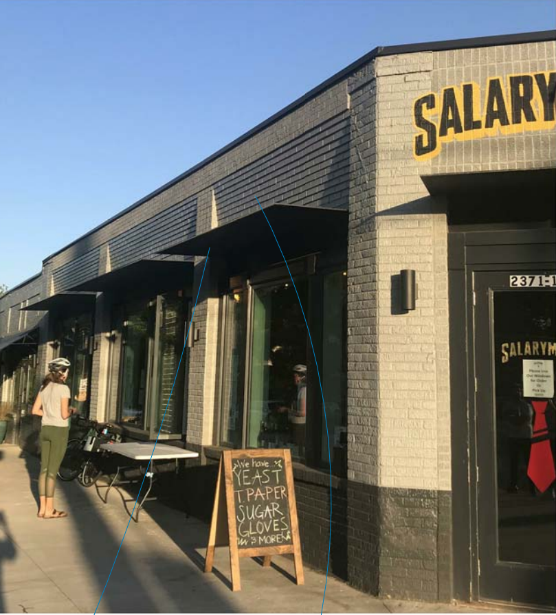
TRADITIONAL BRICK CORBELING DETAILS & STEEL PLATE AWNINGS
