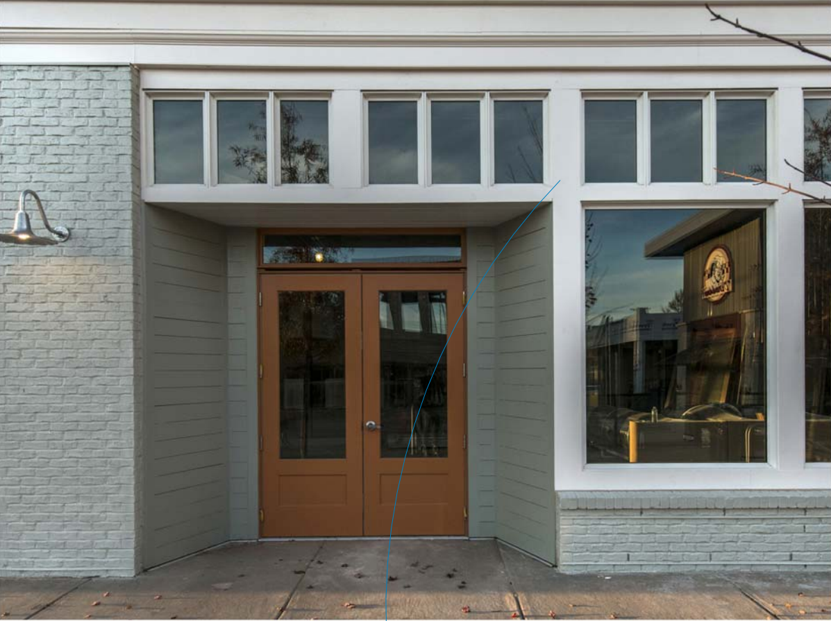
TRADITIONAL STOREFRONT STYLE WINDOWS
