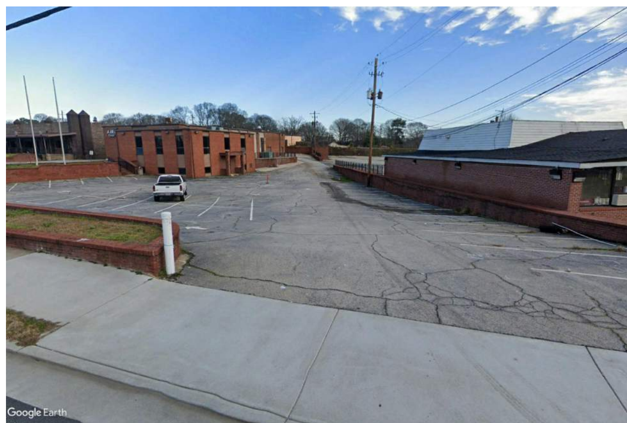
C - NORTH STREET VIEW - NORTH CENTRAL AVENUE
