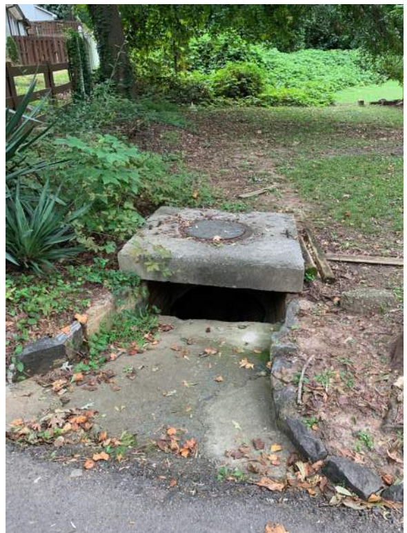
Existing Storm Catch Basin along Lake Avenue
