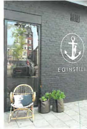
PAINTED BRICK FACADE
