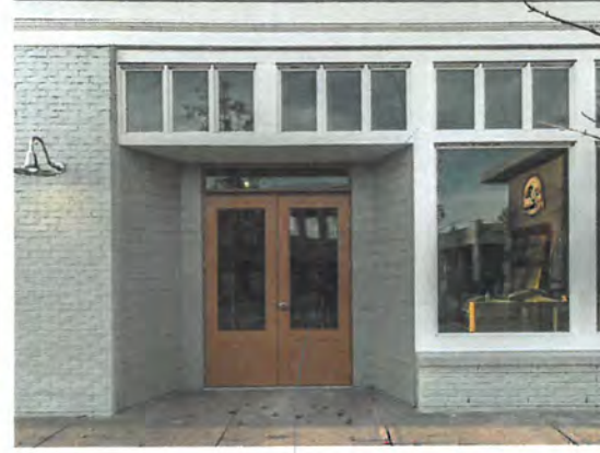
TRADITIONAL STOREFRONT STYLE WINDOWS
