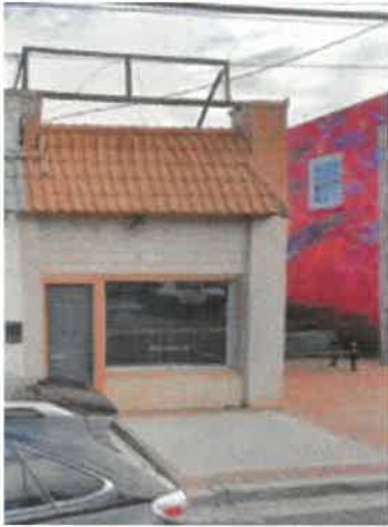
Current Exterior Front 585 N Central Ave. Attached row-house style. End
