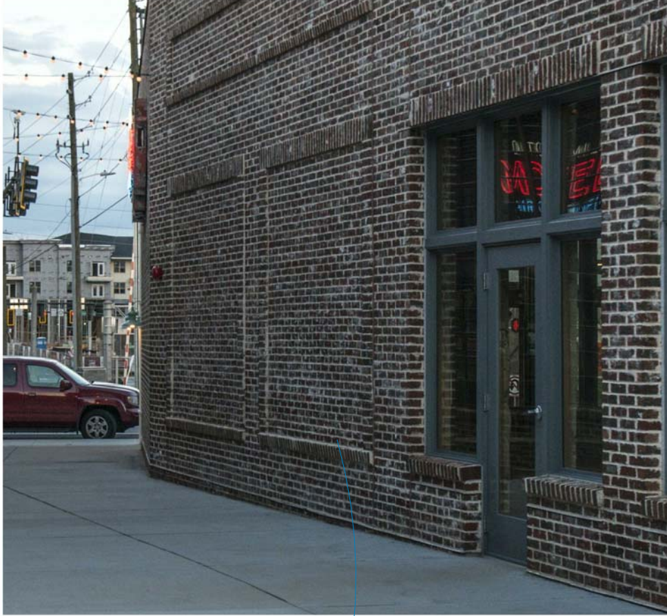
TRADITIONAL BRICK DETAILING TO FRAME ARTWORK
