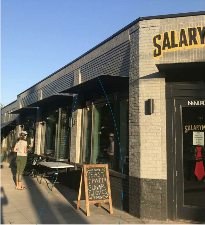
TRADITIONAL BRICK CORBELING DETAILS & STEEL PLATE AWNINGS
