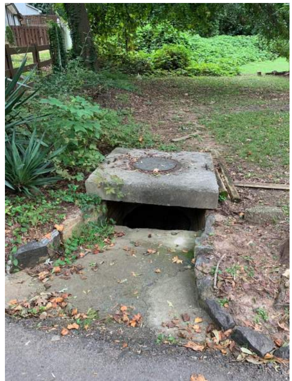
Existing Storm Catch Basin along Lake Avenue
