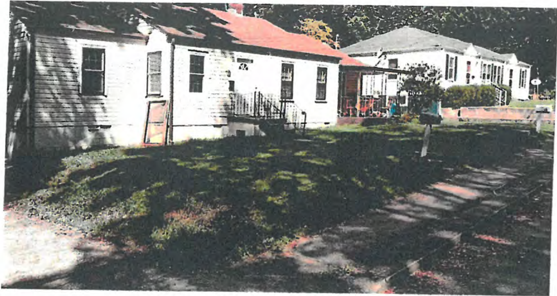
Before pics showing steep embankment on side of home
