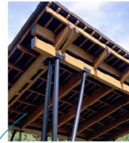
STEEL SADDLE CONNECTION
